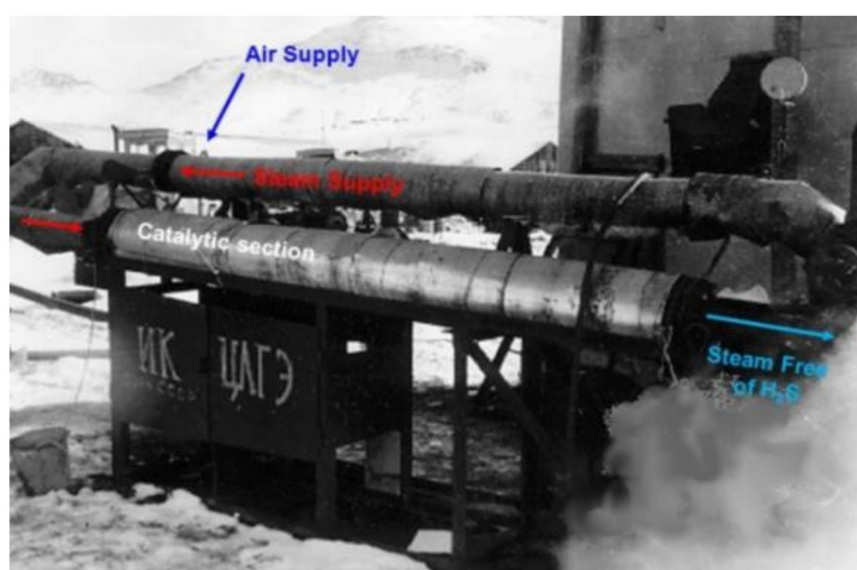
Figure 18. Pilot plant for H_2S removal from geothermal steam.
