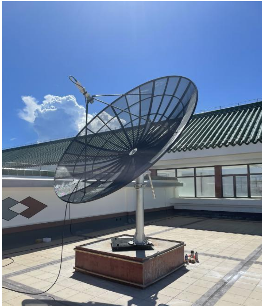
Figure 1. Compact near real-time Himawari-8 satellite data receiving antenna on the roof of Haiqin #2 building of Zhuhai campus of Sun Yat-sen University, Guangdong Province, China.
