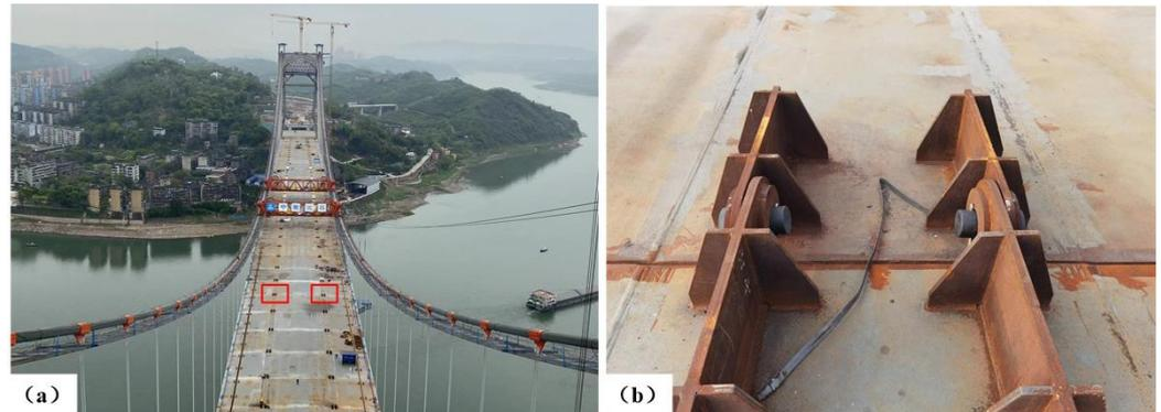
**Figure 5.** Stiffness beam hinge joint method of the Guojiatuo Suspension Bridge. The red box in (a) shows the connection component; (b) shows the enlarged details of the connection component between two stiffness beam.
