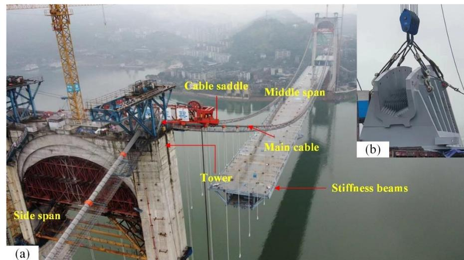
**Figure 2.** Main components of the Guojiatuo Suspension Bridge upper structure. (a) Cable saddle and tower. (b) Enlarged detail of the cable saddle.
