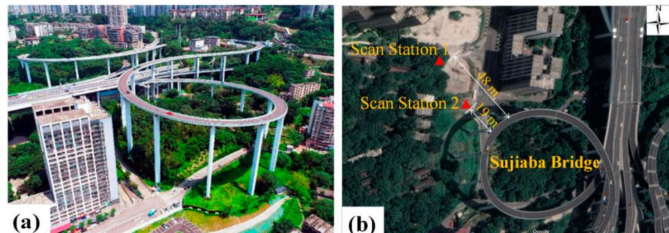
**Figure 5.** Photos showing Sujiaba Bridge. (a) UAV image of Sujiaba Bridge; (b) the schematic diagram of scan station in Sujiaba Bridge and the background is from Google Maps. The scan station 1 is 48 m away from the bridge and station 2 is 19 m away from the bridge.
