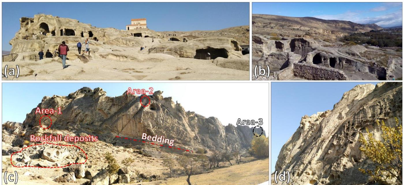
**Figure 4.** The Uplistsikhe cave town complex: top of the rocky terrace with the brick church (a); examples of cave systems and defensive walls (b); the unstable rock cliff bordering the site (red dashed circles highlight April 2019 detachments, Areas 1–2, the black circle the one from July 2019, Area 3) (c); examples of sandstone wind weathering (corrasion) (d).
