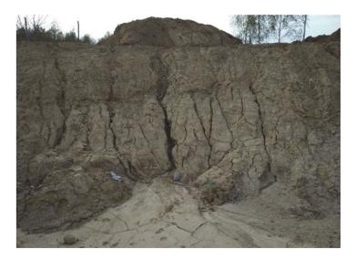
Figure 3. Rills and gullies caused by surficial runoff in silty soil as seen on-site.
