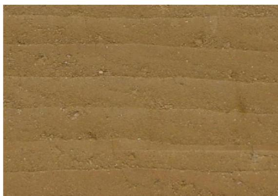
Figure 3. Inhomogeneity of a rammed-earth (RE) wall.
