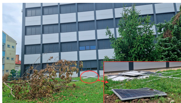
Figure 3. The PV panels were torn off the roof of the Technical School building in Slavonski Brod, Croatia, by the stormy wind.
