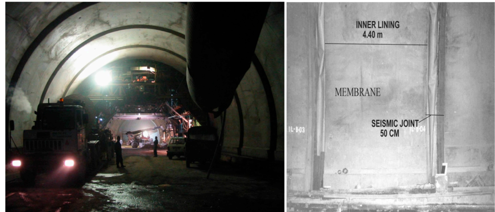
Figure 33. Seismic joints in the inner concrete lining.
