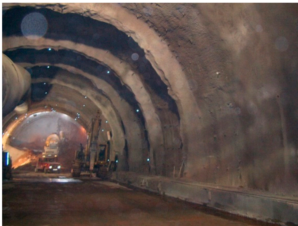
Figure 15. Damage owing to the high deformations in the left tunnel lining (a) and the left tunnel reinforcement works (b) [45].
