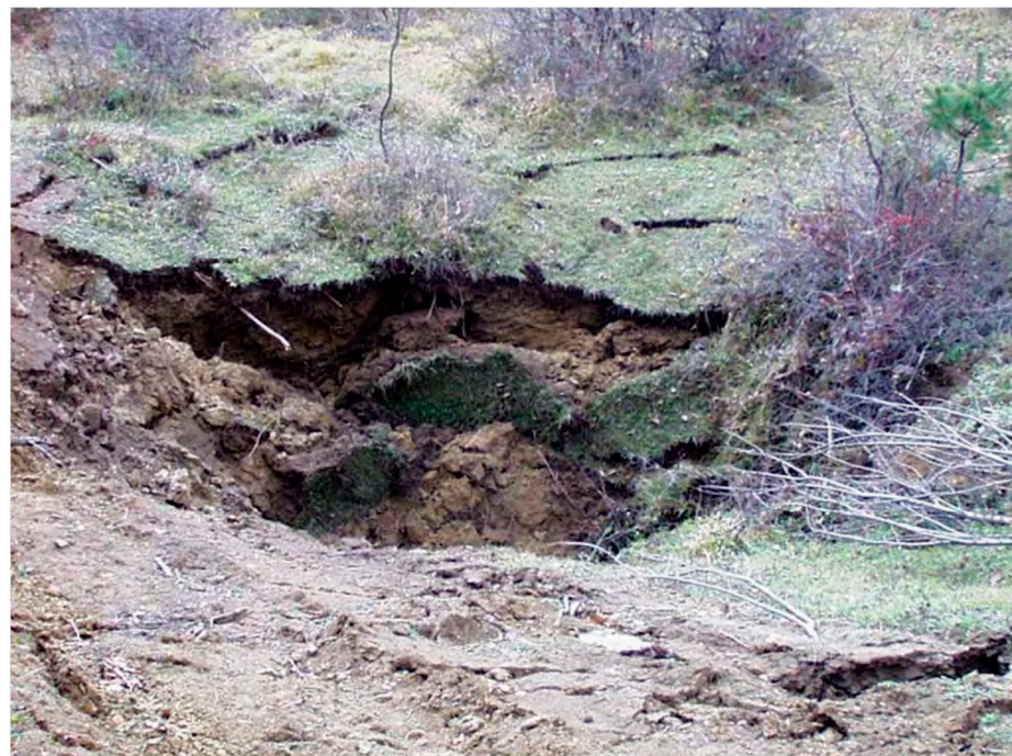
Figure 25. Sinkhole above the tunnel alignment [12].
