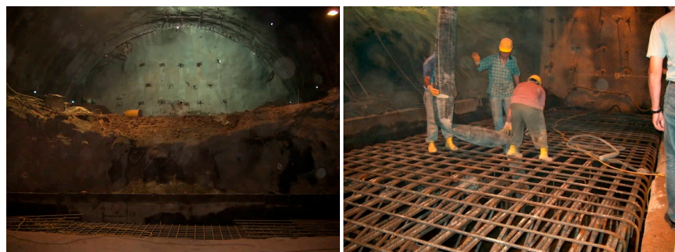
Figure 35. Application of invert with reinforced concrete.
