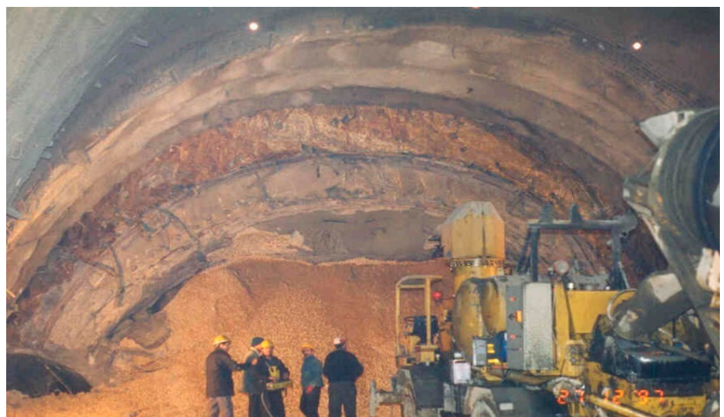
Figure 17. The right tunnel collapse zone between 54 + 147 to 54 + 240 in 1996 (before the Düzce earthquake).
