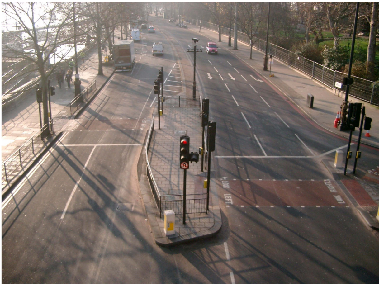
Figure 13. Crossing area with a pedestrian refuge, London, United Kingdom.
