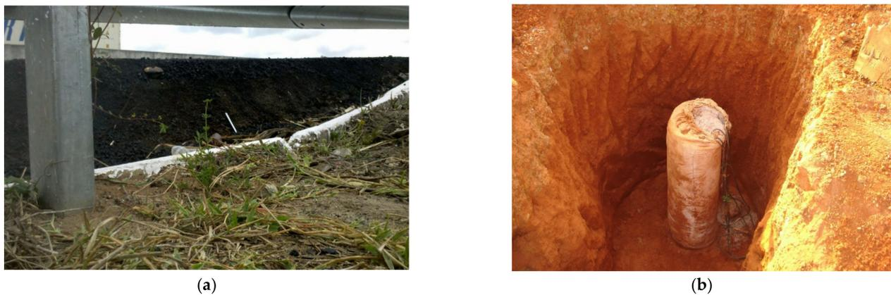
**Figure 7.** Geosynthetic-encased granular columns to stabilise embankments on compressible ground: (a) typical differential settlement between an abutment on soft ground and a bridge; (b) geosynthetic-encased granular column.
