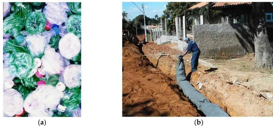
**Figure 21.** Alternative drainage system with a core of compressed PET bottles (images courtesy of H. Paranhos): (a) compressed PET bottles; (b) geocomposite for drainage formed by compressed PET bottles enveloped by a geotextile filter in a drainage trench.
