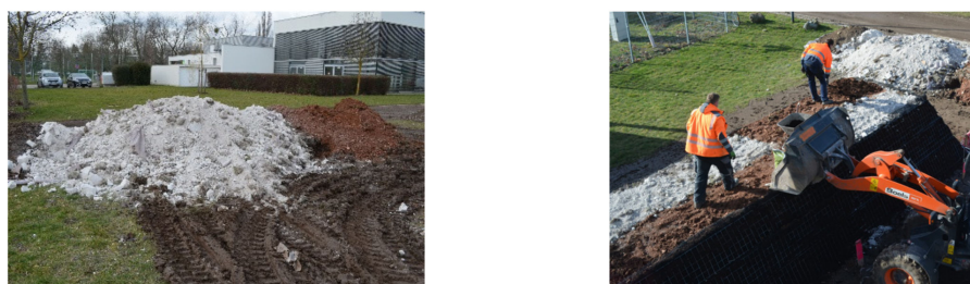
Figure 2. SBM mixed with organic soil, left: before installation, right: after installation in a pilot application. Pictures: Schneider.
