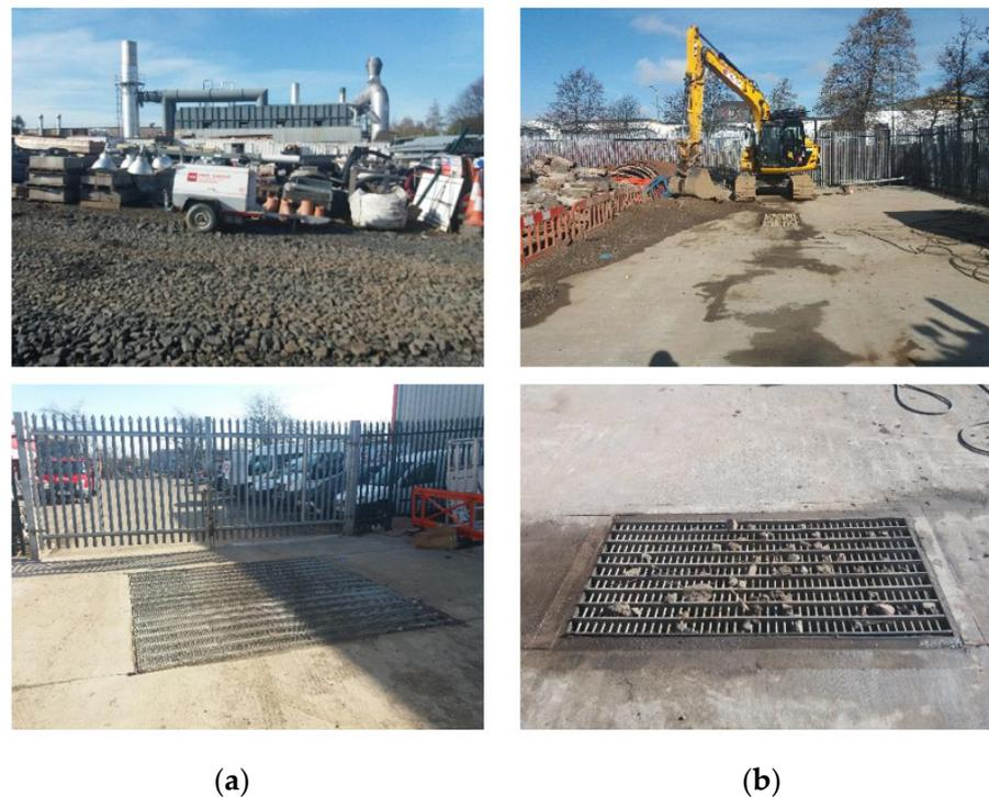
**Figure 6.** Views of storage yard: (a) silt trap at the entrance, (b) vehicle wash area.
