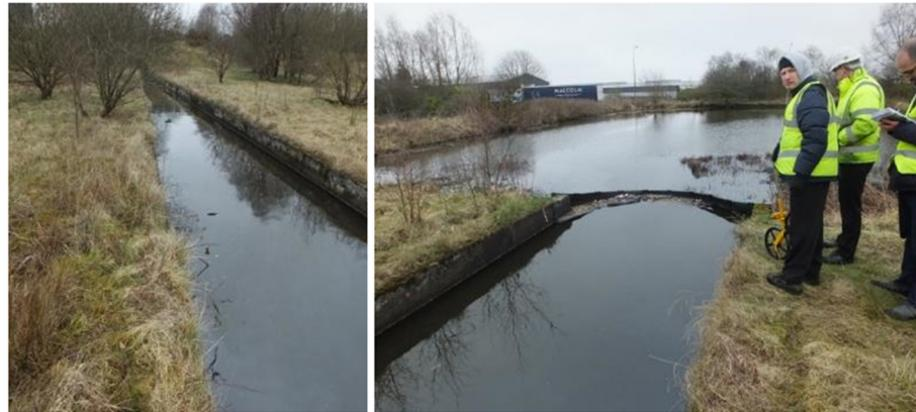
**Figure 13.** Inlet channel to the primary pond and oil boom at discharge into that pond.
