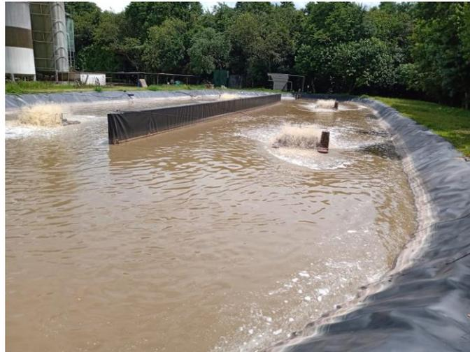
**Figure 1.** Sewage treatment aeration pond under operation.
