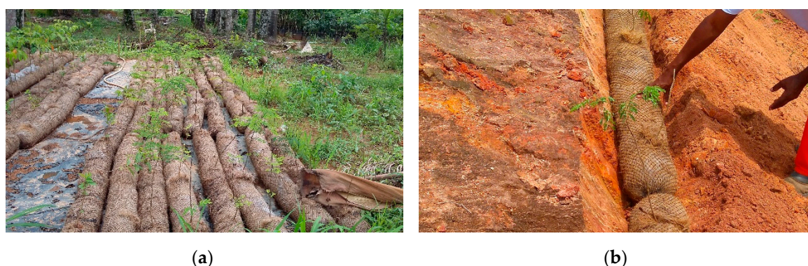
Figure A3. Organic sediment retainers associated with live elements (L-OSRs): (a) storage in the experimental units; and (b) installation of the elements in manually excavated trenches.
