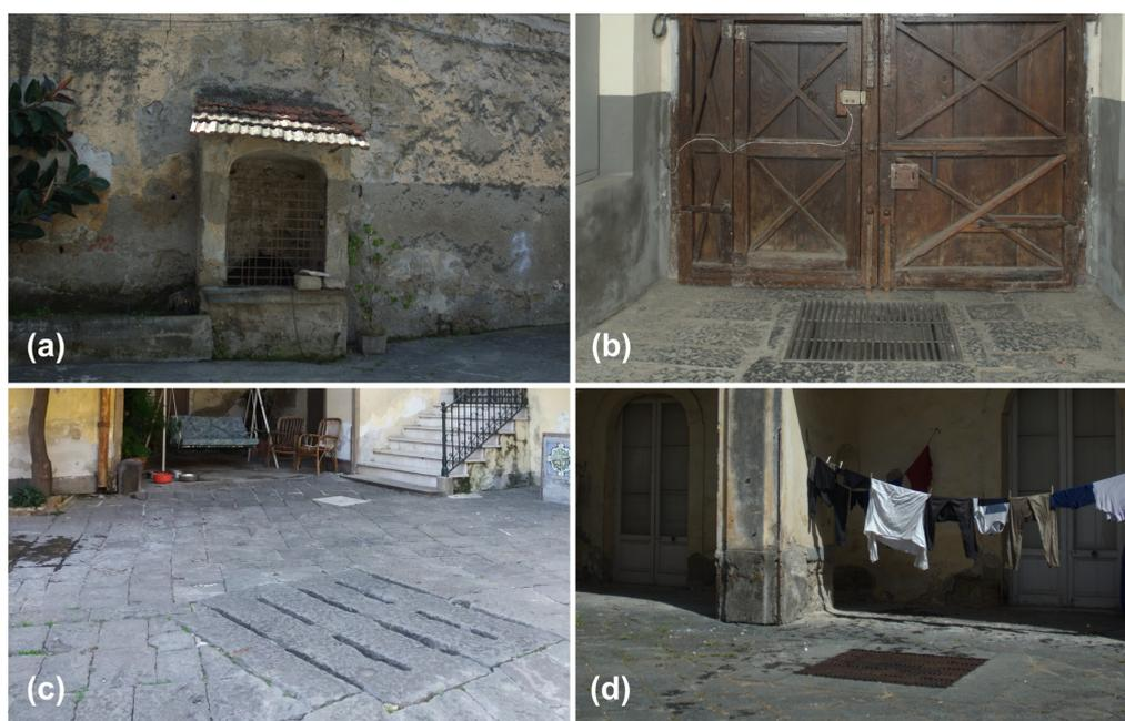
**Figure 11.** Indirect evidence of the presence of underground cavities: (a) buried well; (b–d) large iron and concrete grates (1 m wide on each side).
