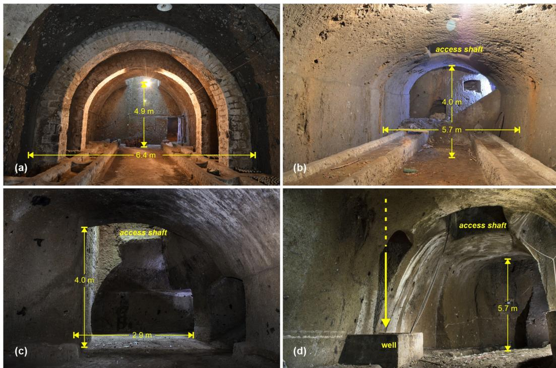
**Figure 6.** Some architectural types of arches of the vaults: (a) semicircular arch; (b) segmental arch; (c) rampant arch; (d) trapezoid-shaped arch.
