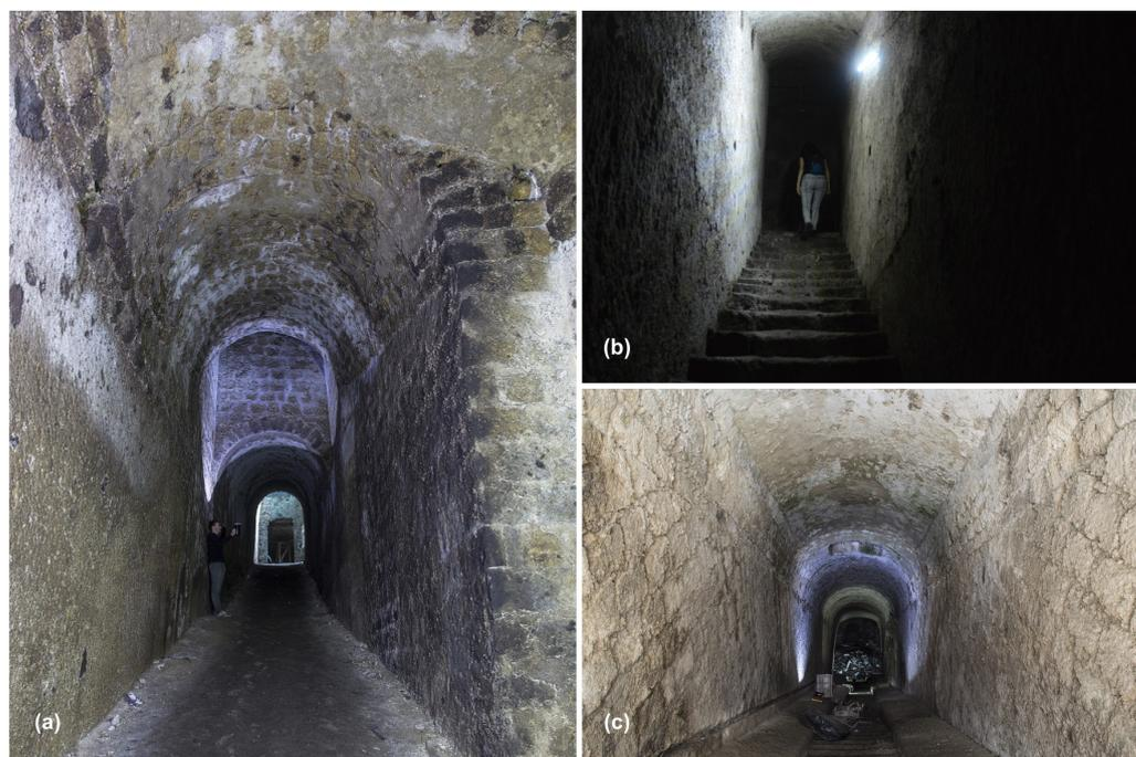
**Figure 7.** Access type: (a) incline ramp, (b) “L”-shaped stairs, (c) straight stairs with slides (1.5 m wide).
