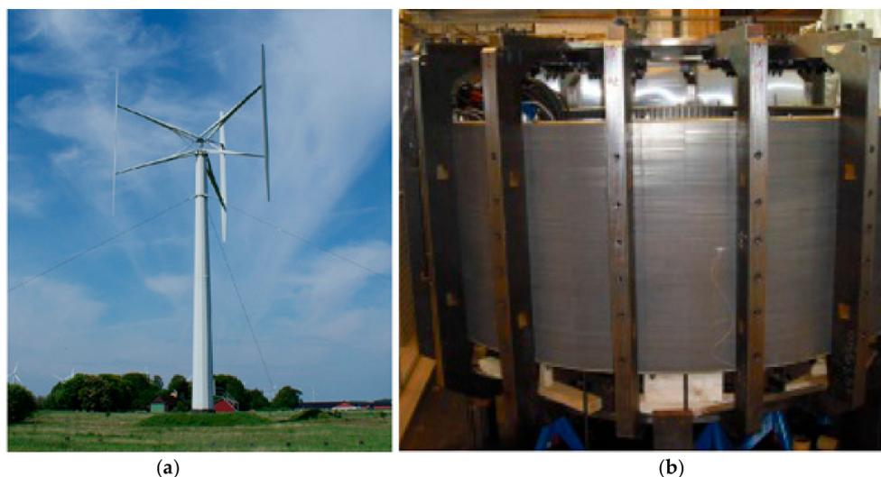
**Figure 13.** (a) Vertical Wind 200 kW (b) Synchronous generator for H-rotors, [56]. Photo by Erik Möllerström. All rights reserved.
