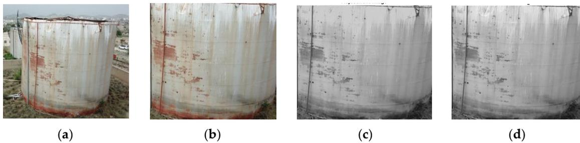
**Figure 4.** Image cropping and resizing: (a) Original image of the whole tank captured by the UAV (b) the image after implementation of cropping and resizing operation (c) the image after conversion process from RGB to gray (d) the image after adjustment.
