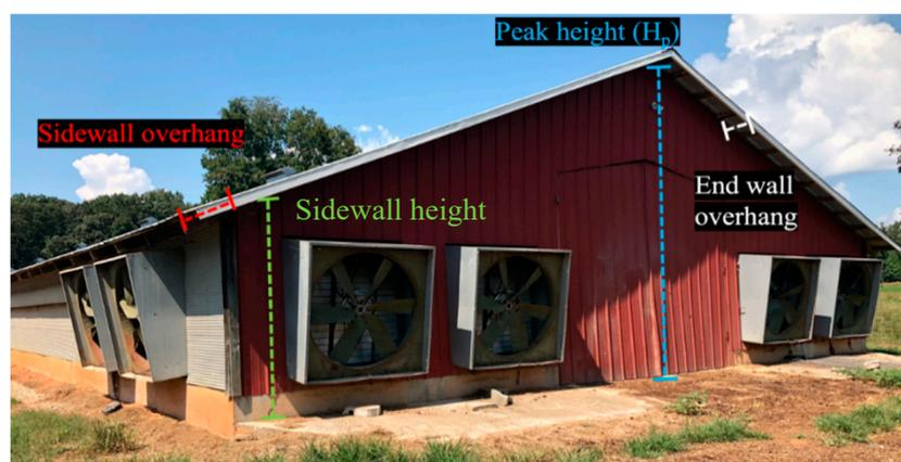
**Figure 3.** Poultry end wall illustrating the location of sidewall and peak height measurements and building overhangs.
