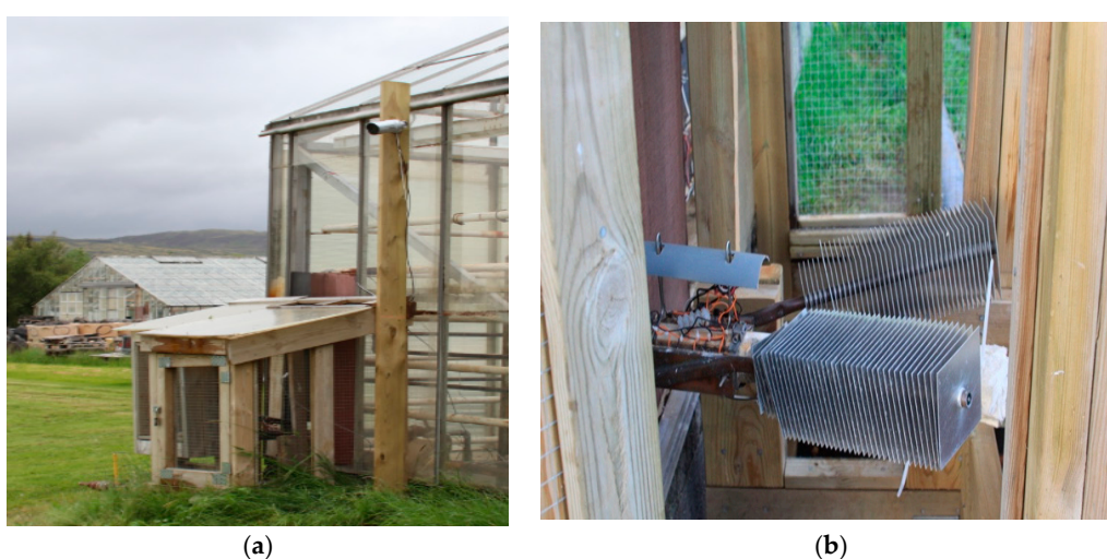
Figure 2. At the Agricultural University of Iceland near Hveragerdi, (a) two co-joined exterior sheds were attached to a greenhouse to enclose and protect the three thermoelectric generators (b) two generators in the first shed.
