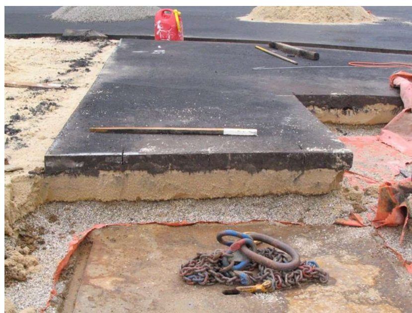
Figure 2. 2004 Melbourne Commonwealth Games temporary track pavement profile.
