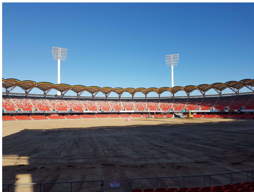
Figure 3. Stripped surface of Carrara Stadium prior to reshaping.
