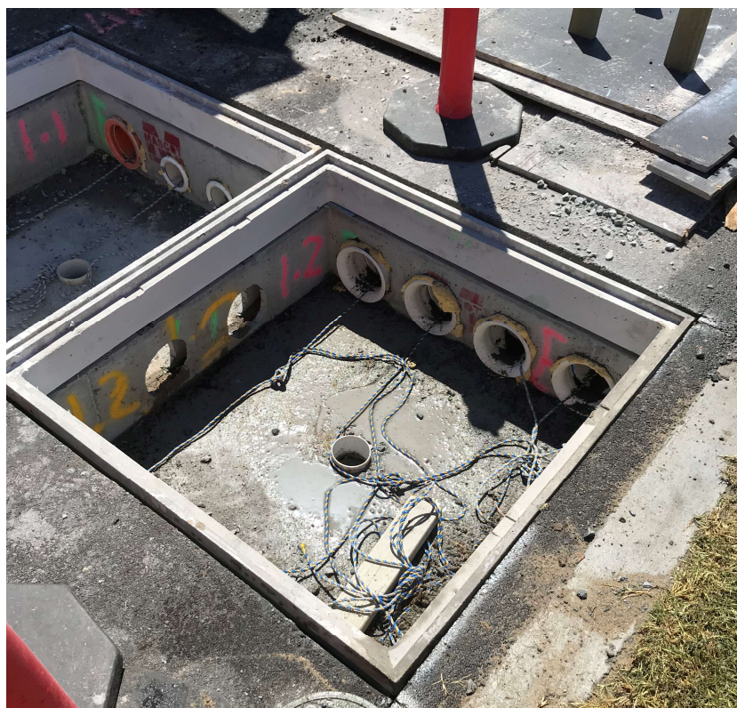
Figure 7. Mechanically protected shallow in-ground service conduits and pits.
