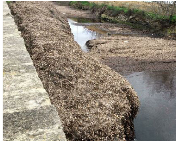
Figure 4. Posidonia Oceanica leaves which obstruct the drains. Original picture by LeccePrima graphically modified for editorial purposes.
