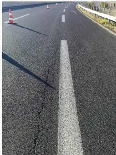
**Figure 16.** Longitudinal crack at location A4 three years after the experiment.
