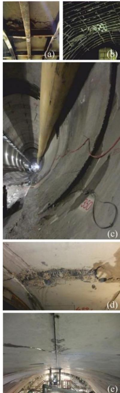
**Figure 7.** Damages on the segments and the reinforcement with NPI profiles (a,b); additional supports; steel-beam, wire mesh, and fiber-concrete shotcrete (c); an example photograph representing excessive plastic deformation in the tunnel (d); an example view of a longitudinal joint in the tunnel (e).
