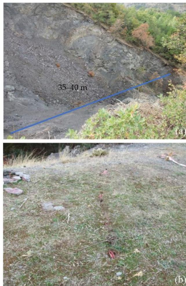
**Figure 6.** View of subsidence developed throughout the TBM excavations (a); tunneling induced surface cracks adjacent to the tunnel alignment (b).
