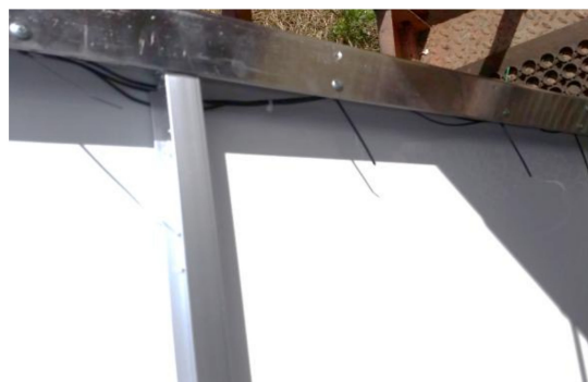
Figure 6. Assembly of the left side aluminum component on the underside of the PV module (top of image shiny silver). All four aluminum components are mounted to the module similarly.
