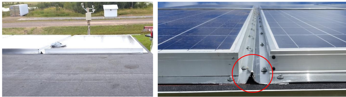
Figure 7. Installation of the first row of adapted PV modules on the bottom of the experimental roof ( left ) viewing from the peak of the roof. The roof felt roof deck protection is shown in the foreground. A bag of screws is shown on the first module for scale. In the background is one of the meteorological stations for the Keweenaw Research Center (KRC) PV systems testing field [35–37]. On the ( right ) is a detail of the overlap between the left and right aluminum components forming a vertical channel. In the red circle the overlap between the two sides is shown. The lip from Figure 3 is shown on the left which covers up the bend from Figure 4 (shown on the right). This creates a waterproof channel connecting the modules in the horizontal plane.
