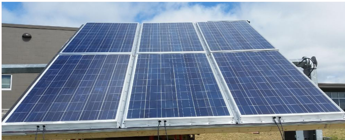
Figure 10. Six module building-integrated photovoltaic (BIPV) roof-mounted test array.
