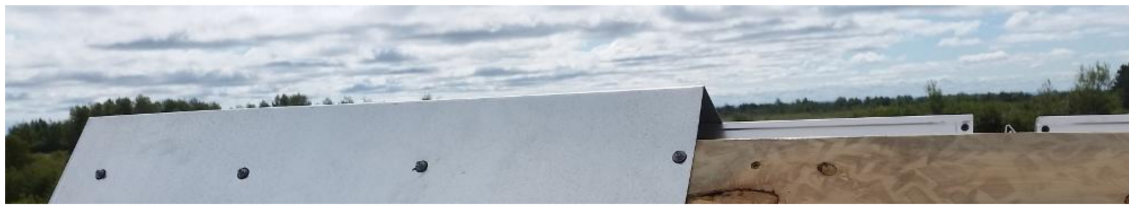
Figure 9. Detail of the final (upper) row of PV modules being covered by an aluminum channel to prevent water intrusion from the top of the BIPV roofing system.
