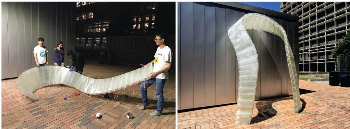
**Figure 19.** Students assemble the 8-m-long, curved sandwich strip of the pavilion in full scale.
