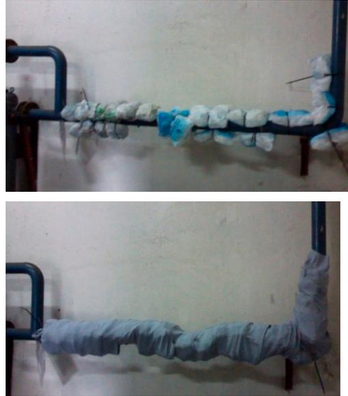
**Figure 7.** Part of the refrigerated installation with ice bags to reduce temperature, from [17], with permission.
