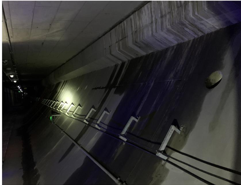
**Figure 1.** Photo of tunnel leakage.
