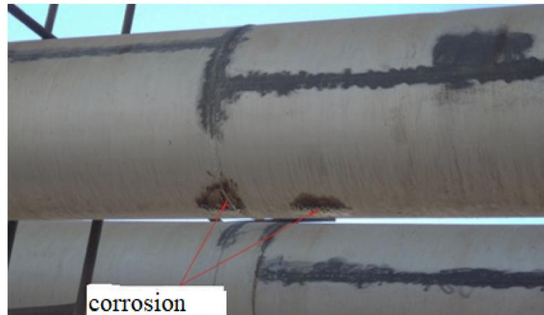
**Figure 1.** Pores in the pipes at the top of the distillation column (photo by Timur Chis).
