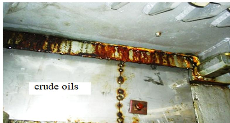
**Figure 2.** Corrosion in the reflux vessel (photo by Timur Chis).
