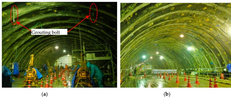
**Figure 17.** The effect of the new grouting method. (a) The grouting process; (b) the effect after grouting.
