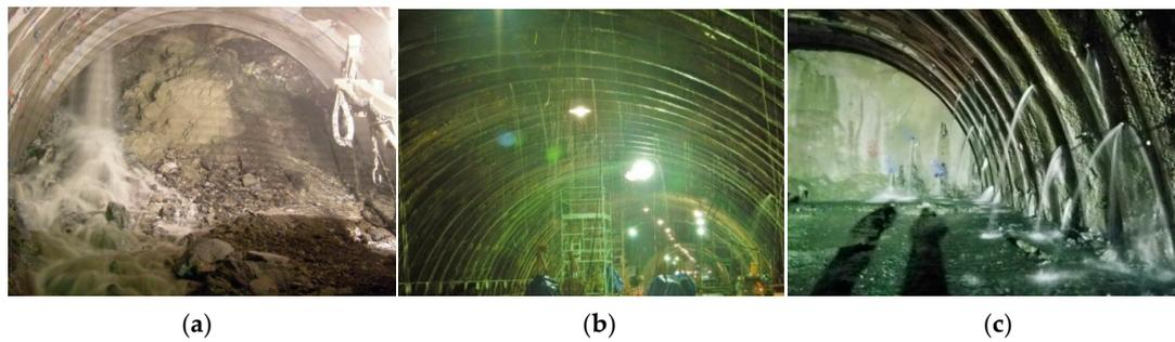
**Figure 4.** Leakage problems during the tunnel excavation: (a) Sudden water inrush during tunneling; (b) Groundwater inflow and water drops; (c) Gushing water in the tunnel.
