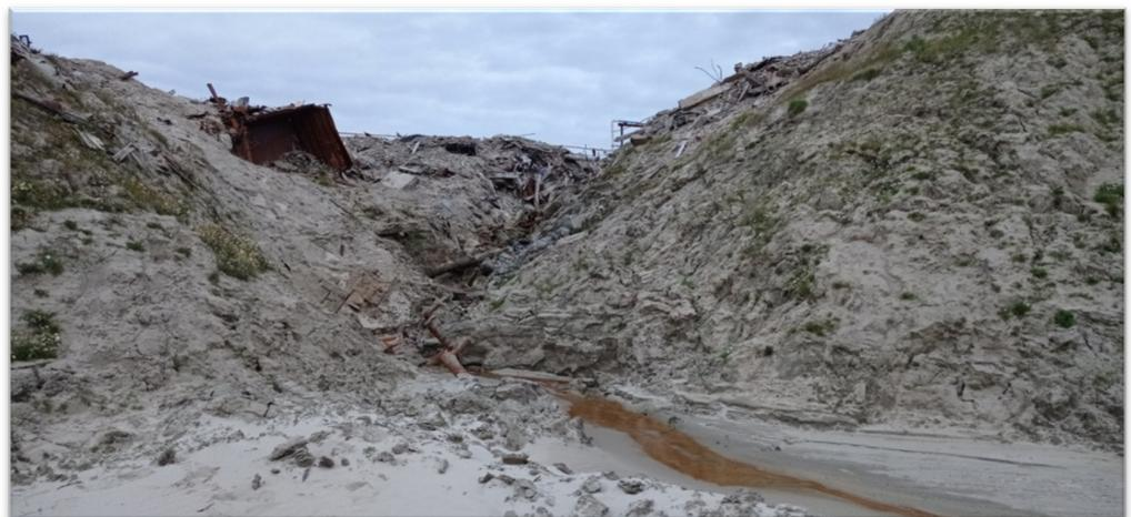
**Figure 5.** Construction waste used to stop gully development. Photos by D. Bogatova.
