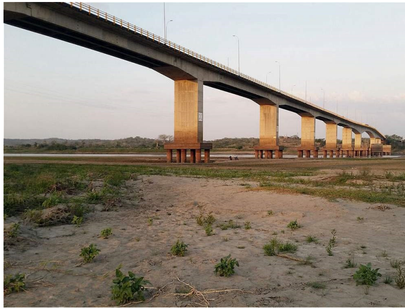
Figure 10. Evidence of riverbed incision at Plato—Zambrano bridge, lower Magdalena downstream of Tacamocho (see Figure 8 upper border) [50].
