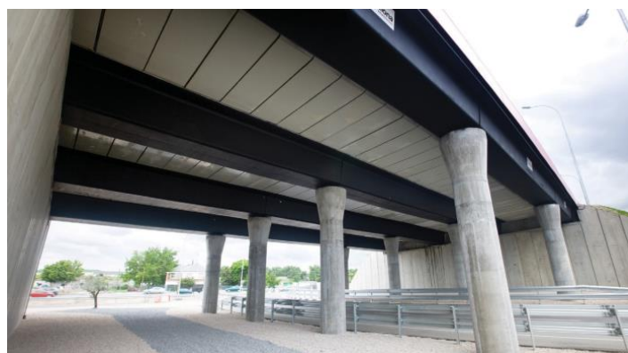
Figure 17. M111 road bridges, Madrid, Spain, consisting of moulded FRP primary beams and concrete deck, were built in 2007 [65,68].
