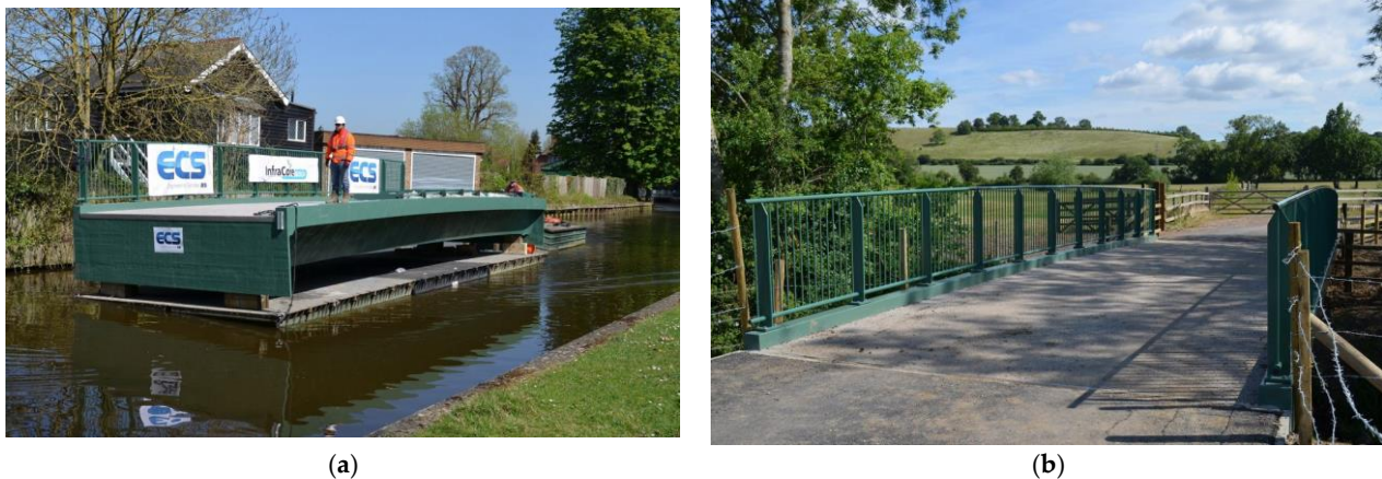
Figure 21. Mapledurham Footbridge, Mapledurham, Oxfordshire, UK, built in 2015 [8]: (a) FRP bridge deck delivered to site by floating on a barge along River Thames; (b) Mapledurham FRP bridge installed with no physical joints.
