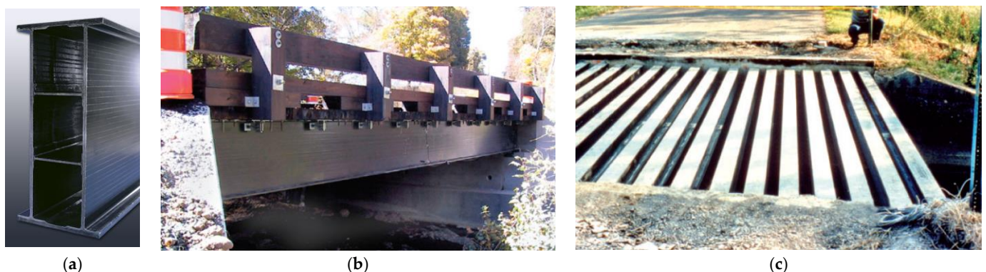
Figure 35. Pultruded FRP highway bridge girders [101]: (a) Strongwell EXTERN DWB; (b) Route 601 highway bridge in Sugar Grove, Virginia, USA using EXTERN DWB 900 × 450 mm, built in 2001; (c) Tom's Creek Bridge, Blacksburg, Virginia, USA, built in 1997 and used EXTERN DWB 200 × 150 mm.
