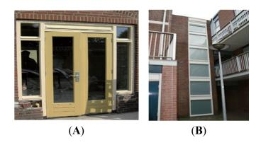
Figure 11. Acetylated radiata pine door (A) and windows (B) that were installed in Japan 2008.
