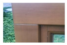
Figure 6. Corner window joint in an acetylated window.
