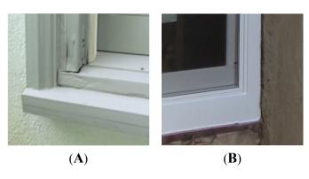
Figure 8. Decay in the corner of a control window after three years (A); no swelling or decay in the acetylated window after five years (B).
