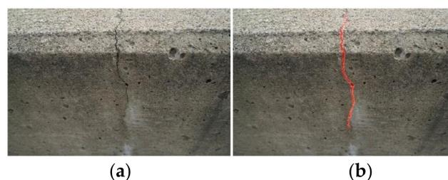
**Figure 10.** Comparison of original DeepLabv3+ and Dense-DeepLabv3+ crack segmentation results. (a) original image (b) Dense-DeepLabv3+.
