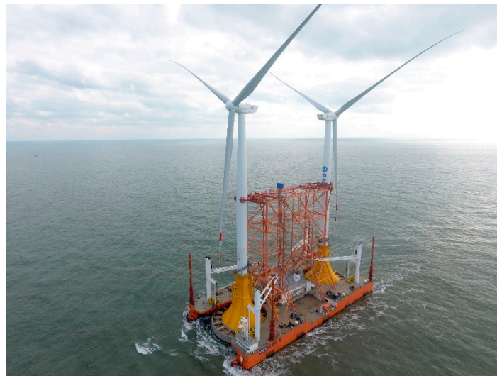
Figure 1. Composite bucket foundation for offshore wind turbines (photo was taken by the author).
