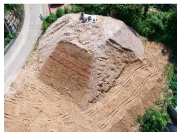
**Figure 4.** Construction of the model slope.
