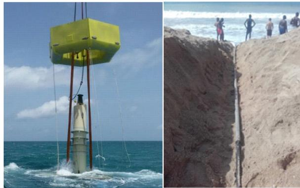
**Figure 9.** A WEC deployed together with the buoy (**left**) and the connection pipe (**right**).
