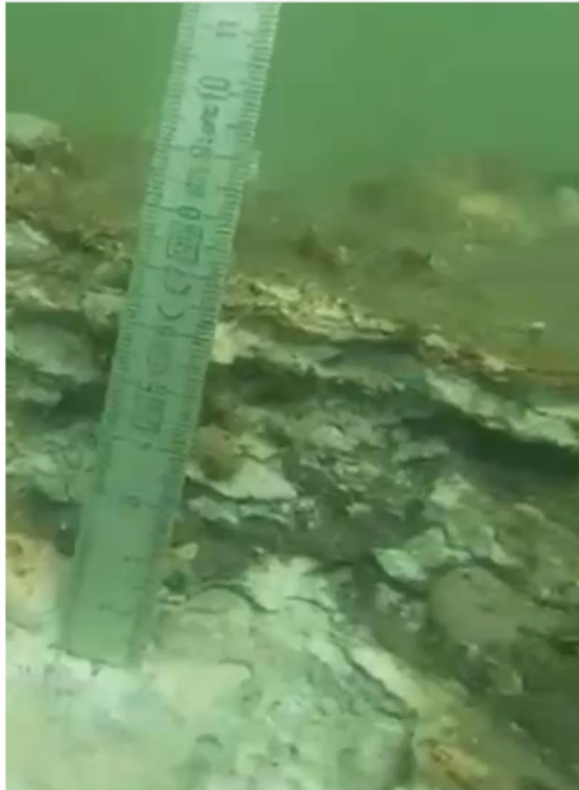
**Figure 11.** External wall deterioration located in Section A3 (it is worth noting that the poor resolution of the image is due to the peculiarity of the subsea environment).
