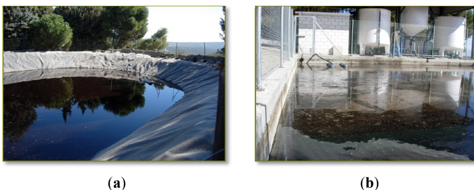
Figure 1. Olives washing wastewater (OWW) (a) and olive oil washing wastewater (OOW) (b) storage and evaporation lagoons.
