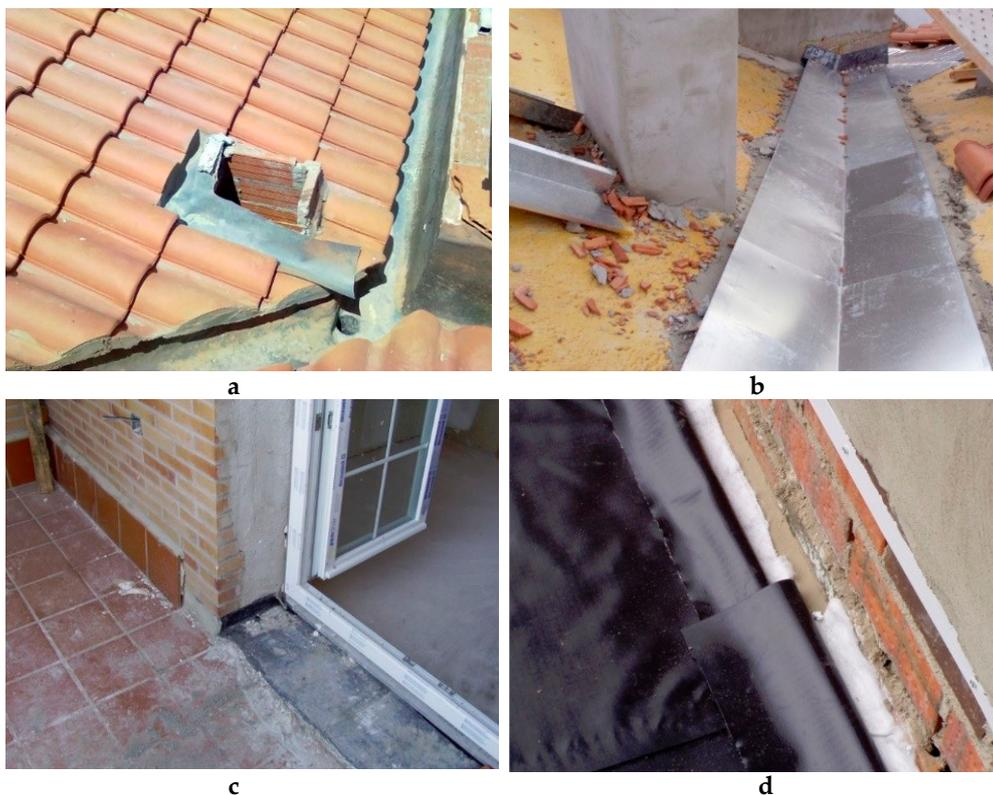
**Figure 9.** Photographic examples of some construction problems in roofs due to design or execution flaws. (a) PITCHED ROOF: Incorrect tail-end between the base of a chimney and ceramic tiles; (b) PITCHED ROOF: Position of a roof hip improperly draining towards a wall; (c) FLAT ROOF: Lack of sufficient height in the access door sill; (d) FLAT ROOFS: Inadequate tail-end of the membrane with the perimeter parapets.
