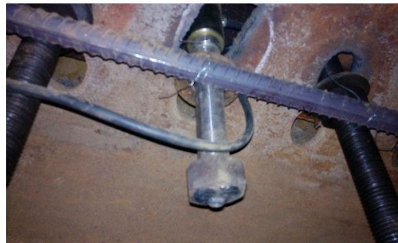
Figure 15. Installation of monitoring sensors.
