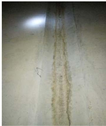
**Figure 15.** Crack on the bottom of the water groove.
