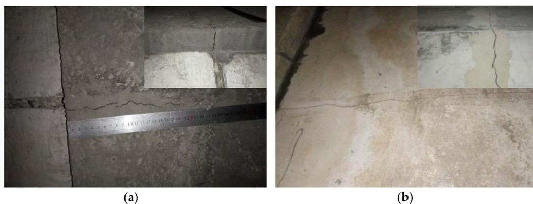
Figure 10. Typical cracking of (a) mastic asphalt waterproofing layer; and (b) concrete waterproofing layer.
