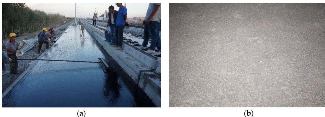
Figure 6. Construction process (a) and completed surface (b) of mastic asphalt waterproofing layer (MAWL).
