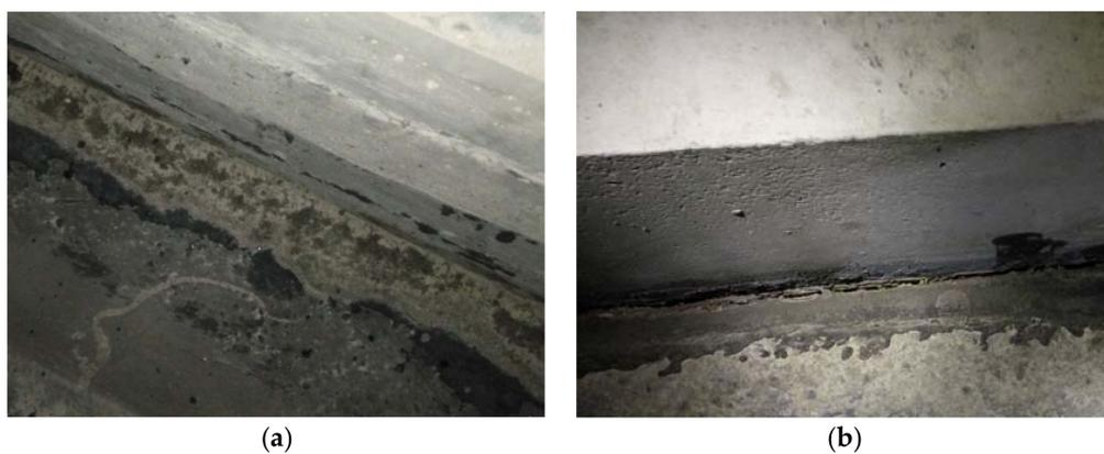
**Figure 12.** Status of construction joint after two years of operation: (a) construction joint in good condition; and (b) local debonding of construction joint.
