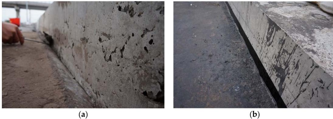
**Figure 7.** Joint treatment process: (a) V-shaped groove; and (b) and grouted joint.
