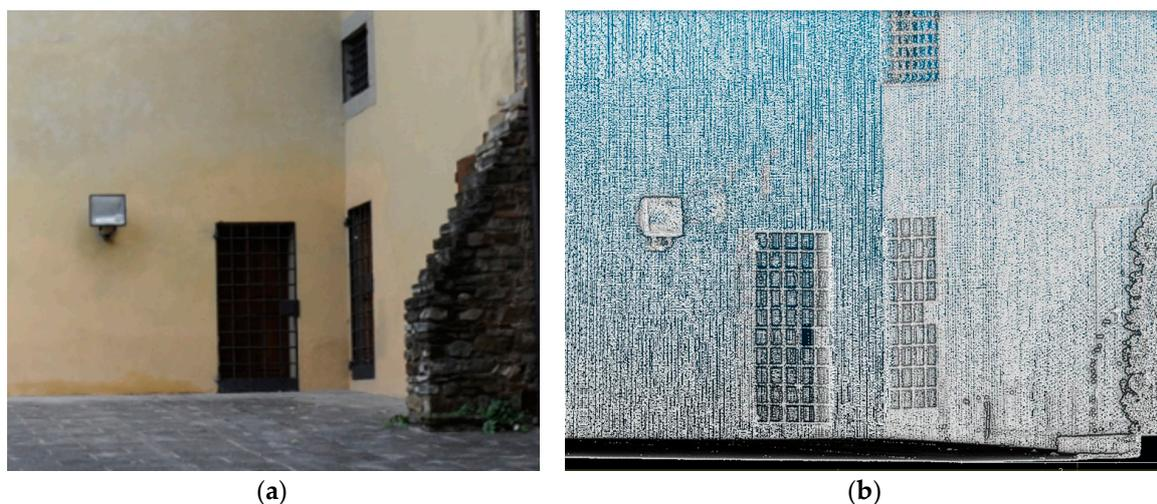
**Figure 19.** Corner of the chosen building for assessing the recognizability of architectural details; (a) photo; (b) reference dataset statically acquired by terrestrial laser scanning (TLS) and down-sampled with 1-cm average resolution.
