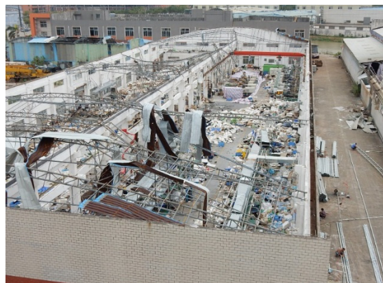
Figure 3. Mainframe collapsed during the typhoon event [6].
