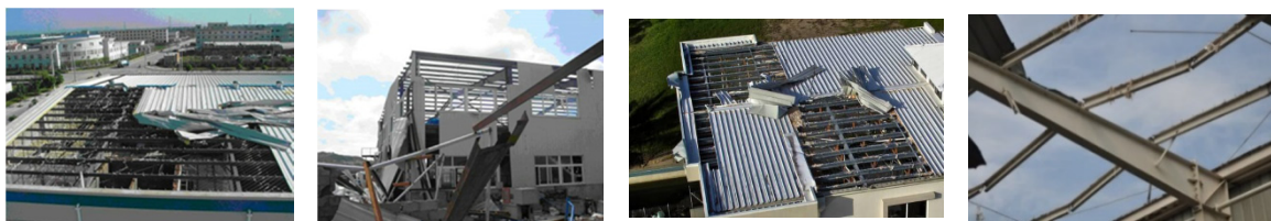
Figure 1. Failure of cladding-fastener connections.
