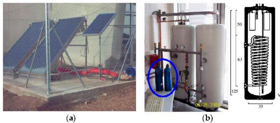
**Figure 3.** (a) Solar thermal collectors (b) Hot-water tanks with PCM modules. Reproduced with permission from [74]. Elsevier: Solar Energy Materials and Solar Cells, copyright 2006.
