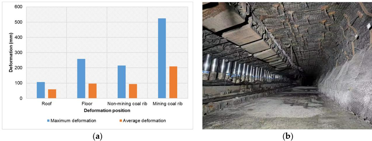
**Figure 11.** The effect of field application in withdrawal roadway 21405: (a) The deformation; (b) A photograph of withdrawal roadway 21405 after mining.
