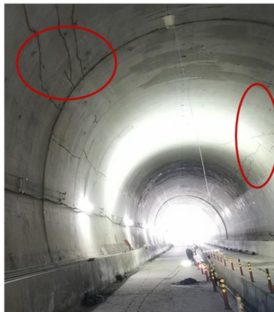
Figure 7. Photograph of longitudinal cracks on both sides.
