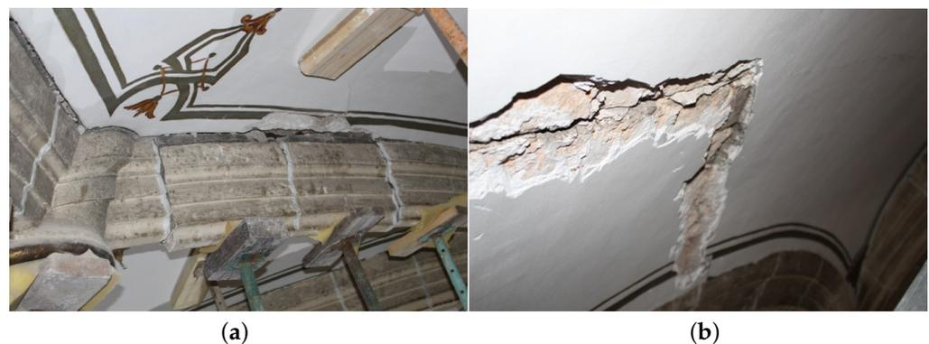
**Figure 15.** (a): Downturned voussoirs of diagonal arches. (b): Deformations and cracks in vaults.
