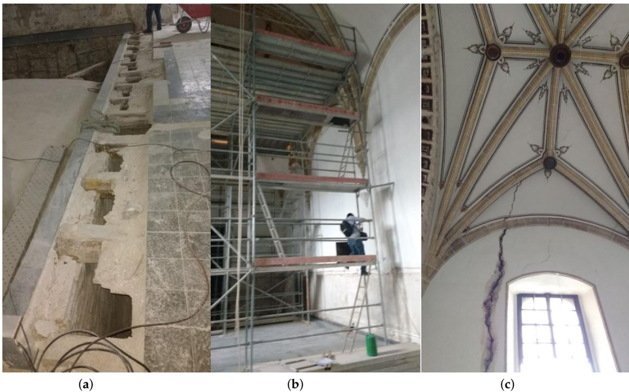
**Figure 3.** Construction process in the restoration. (a) Original slab floor with horizontal wood joists (b) Falsework for stability guarantee in the works (c) the active vertical fracture along wall and vaults disturb stability of the study complex that must be consolidated.
