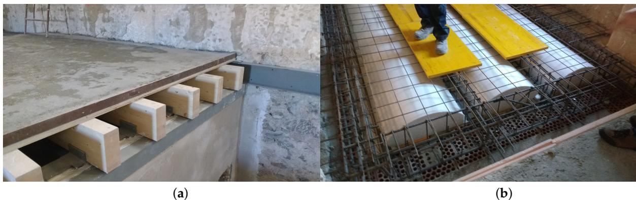
**Figure 4.** (a): Slabs using laminated wood beams. (b): Joists-beam concrete slab built in situ.
