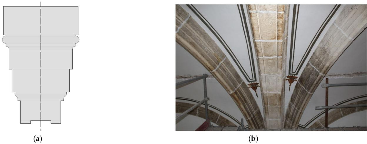
Figure 9. (a): Typical cross-section of the transverse arches. (b): transverse and diagonal arches (in addition to the former arches).
