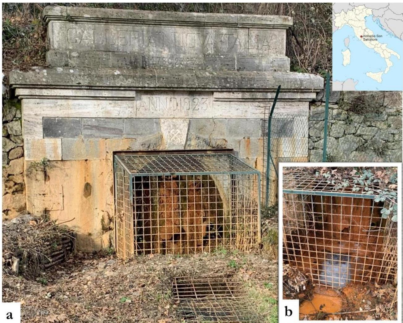
**Figure 1.** Location of Abbadia San Salvatore: (a) Galleria Italia and (b) a detail of the water discharge where the reddish-whitish color can be observed.
